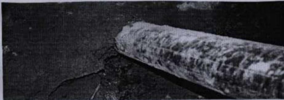
Plate -2- A seepage below the pipe of water drain, where it is entering the pumping station building.
