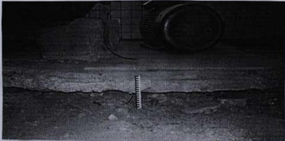
Plate -1- Cavity between the concrete floor and the soil in the high pumping station building.
